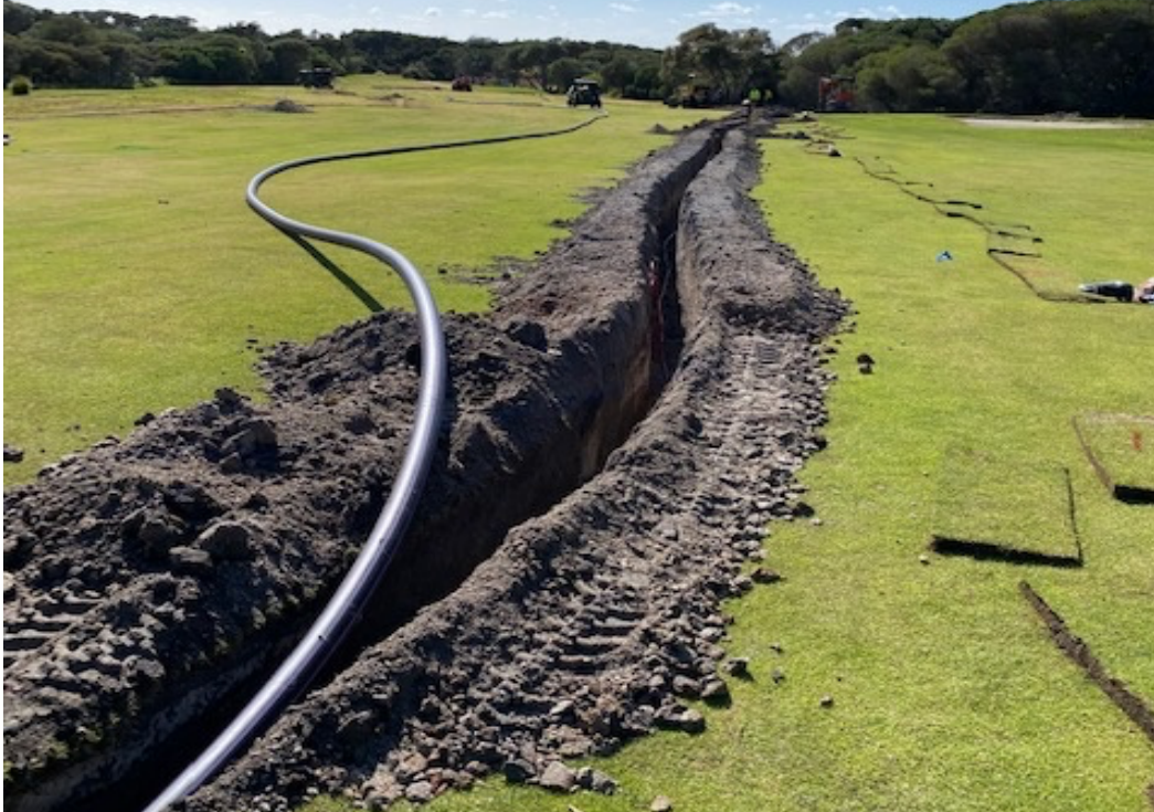
Pictured is the open trenching on the 6 th fairway
